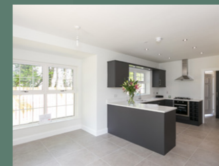
Floor & Wall Tiling
